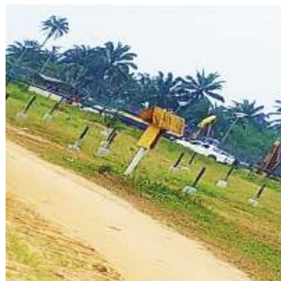
SPDC trunk line showing ground water monitoring wells
