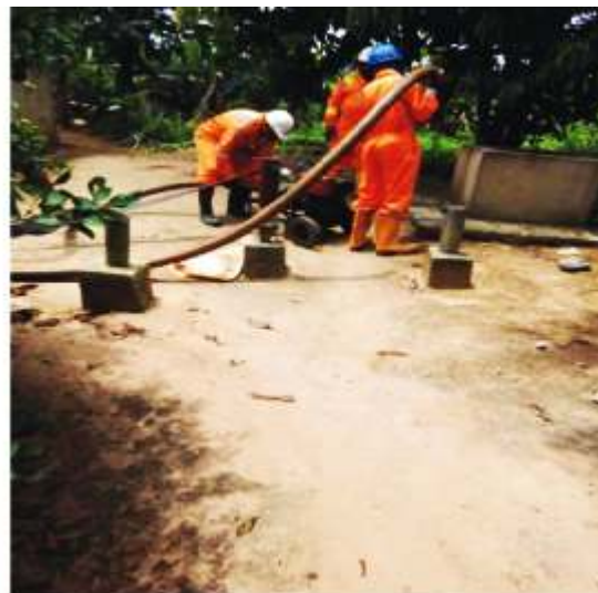
SPDC staffs pumping crude oil from water well
